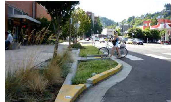
Mid-block crossing, curb extensions, stormwater treatment
