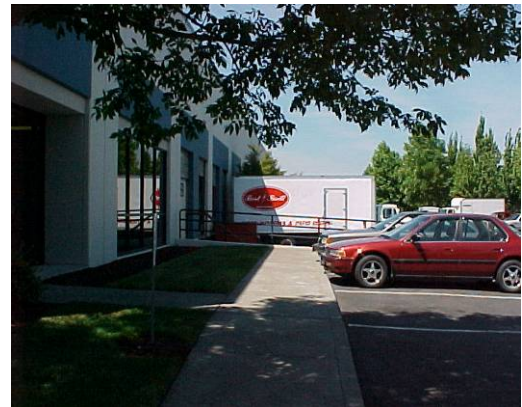
Building functions, like office and loading docks, should be physically separated. Access to office entrance should be convenient and safe.
