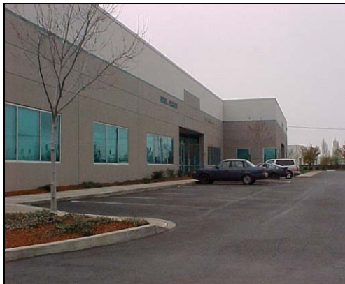
Accent paint and details within the concrete effectively breaks-up the bulk of the facade.
