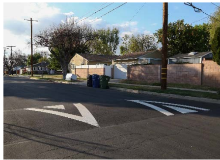
Example of speed hump
