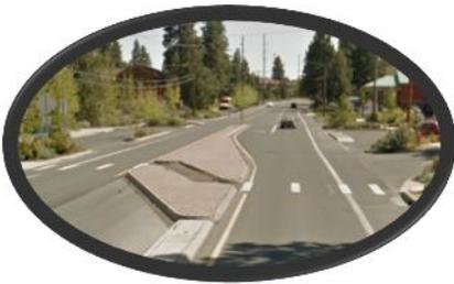
Medians can be used when there are limited gaps in traffic or when there are multiple lanes of traffic to cross in each direction. Oregon Bicycle and Pedestrian Guide notes that medians should be considered the first option on multi-lane, two way roadways<sup>20</sup>.
