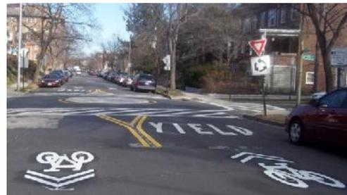
Figure 17 Raised Intersection+Mini Roundabout Speed Management
