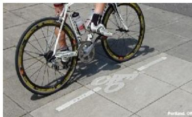
Figure 14 Bike Detection Zone at Signal
